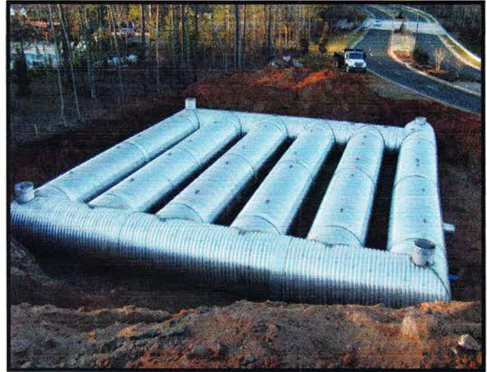
96", 12 gauge Aluminumized Steel Type 2 was utilized for this pre-fabricated underground detention system. Corrosion resistance of AST2 gives designers assurances of a system that will satisfy long service life expectations
