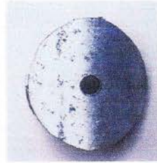
Snohomish County, WA Installed 1952 Inspected 1995
