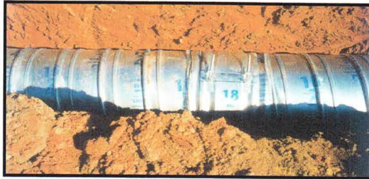
Annular bands ensure that field connections prevent displacement of the pipe due to backfilling operations, fill settlement, or traverse earth pressure.
